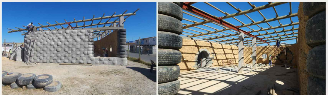
The Building Modality : Used tyres, eco-bricks, film-set waste bricks, and wine bottles
